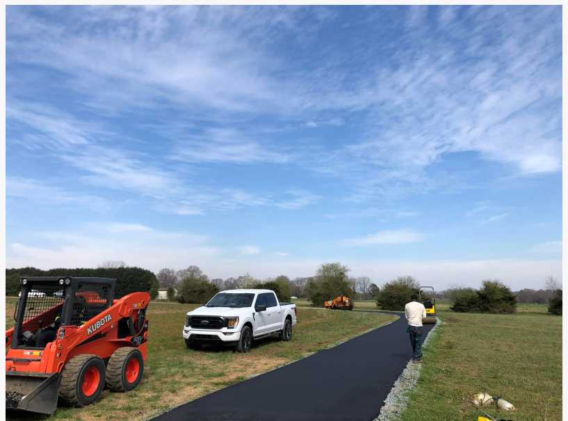
Asphalt Driveway Paving Driveway Repair in Charlotte, NC
