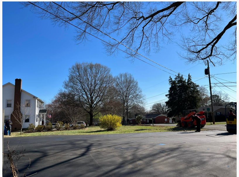
Asphalt Driveway Paving Driveway Repair in Concord, NC
