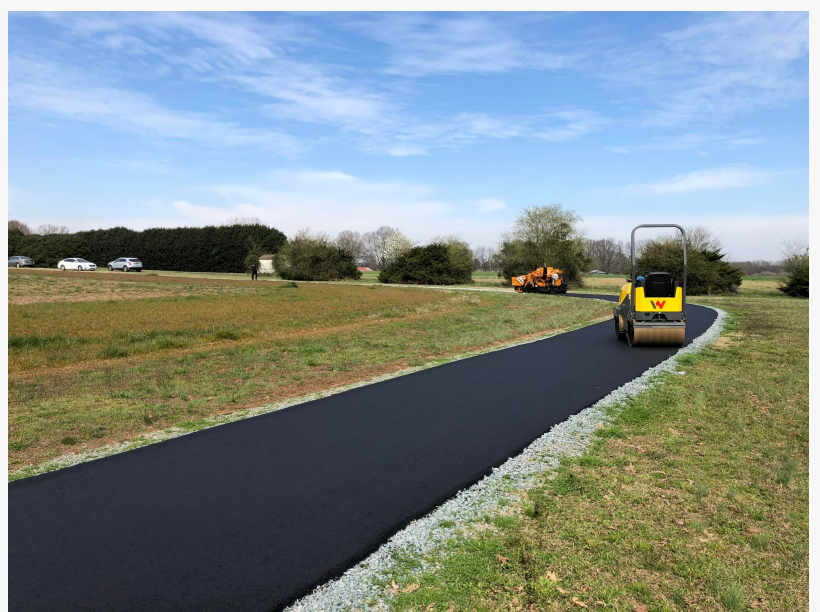
Asphalt Driveway Paving Driveway Repair in Huntersville, NC
