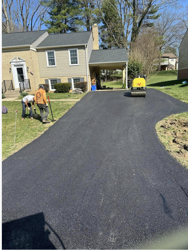
Asphalt Paving Driveway Paving in Gaithersburg, MD
