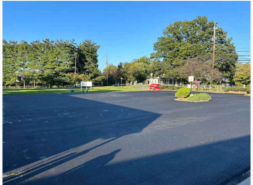
Asphalt Parking Lot Paving Driveway Paving in Rockville, MD
