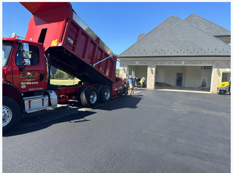
Asphalt Parking Lot Paving Driveway Paving in Potomac, MD
