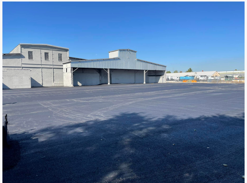
Asphalt Parking Lot Paving Driveway Paving in Urbana, MD
