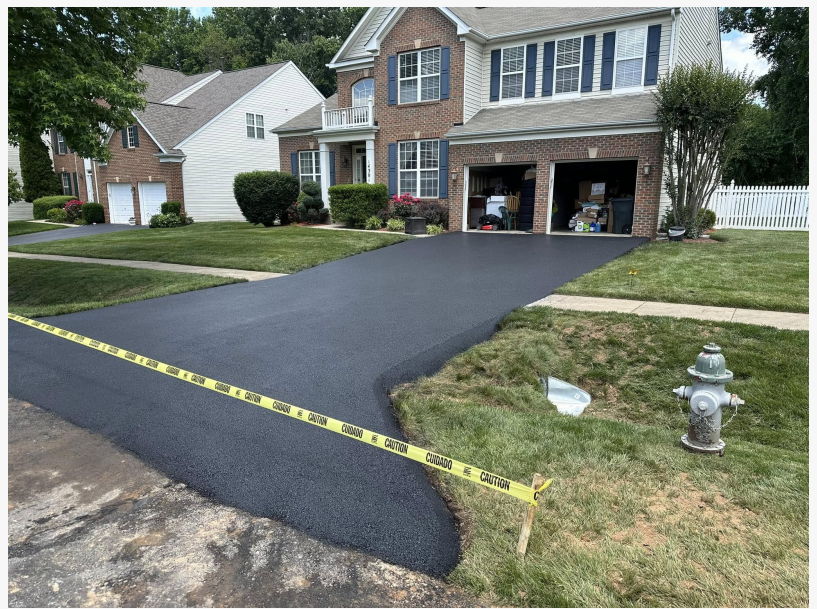
Asphalt Paving Driveway Paving in Frederick, MD
