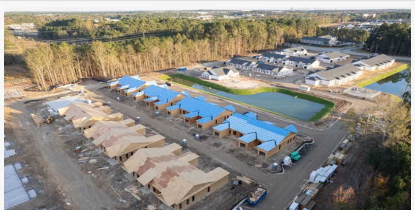
Vertical Construction Underway at Noble Vines in Port Wentworth, Ga.
