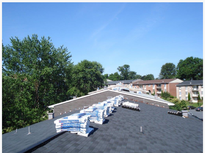
Commercial Roofing in Fort Lauderdale, FL
