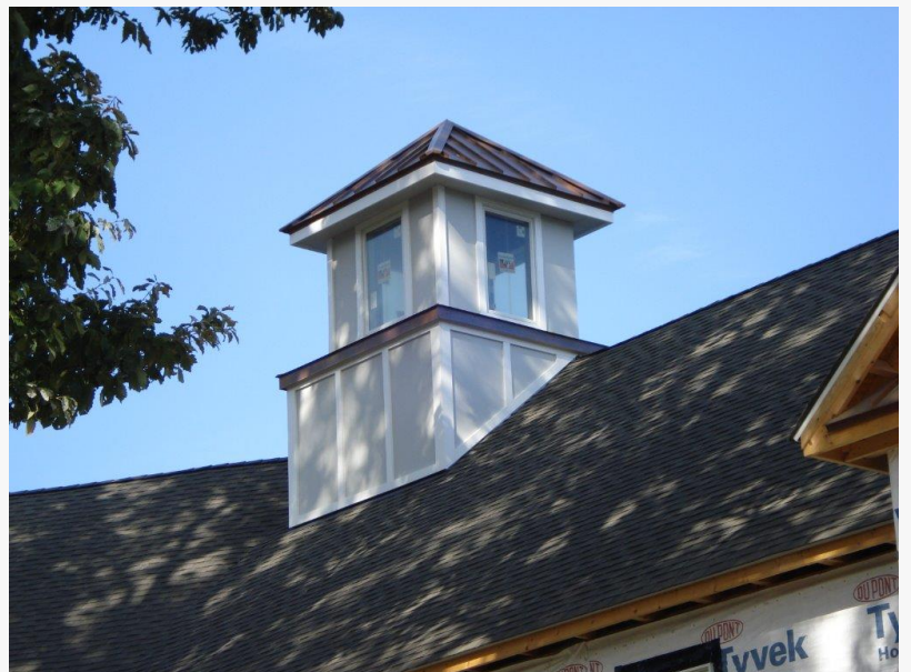
Roofing Company in Hollywood, FL
