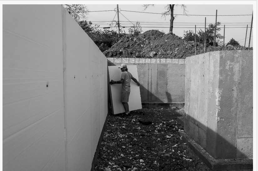
Kala team member installing insulation to the interior of the foundation
