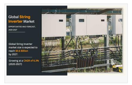
String inverter is a device used to convert the energy generated from the solar panel i.e. direct current (DC) to alternating current (AC) for residential and other AC applications. Solar inverters
