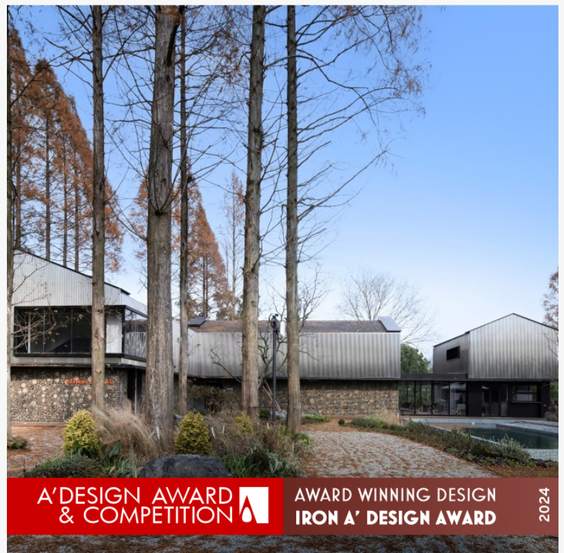
Renovation Of Belight Camp House
