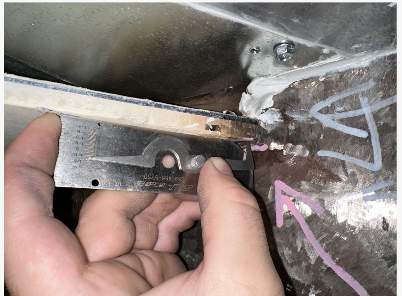
Inspecting for weld undercut with accuracy in Phoenix, AZ..
