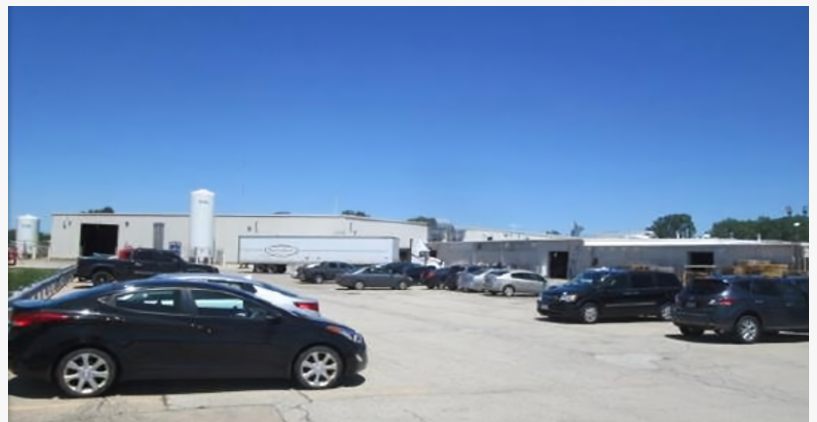
606 East Murdock Avenue facility in Oshkosh, Wisconsin, a 190,000-square-foot industrial property acquired by New Blueprint Partners
