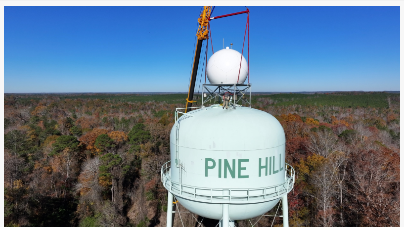
Climavision's X-band radar installed in Pine Hill, Alabama
