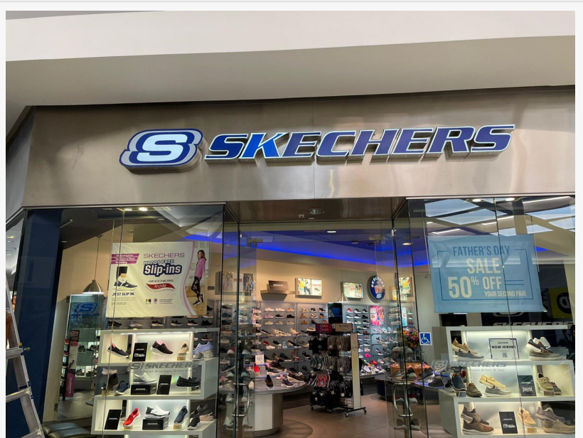
Skechers lighted sign by Royal Signs & Awnings
