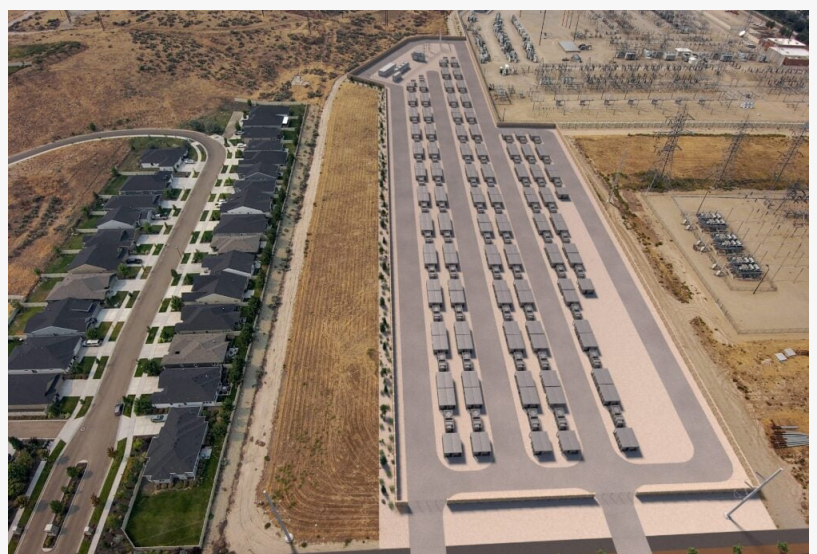
A render of Idaho's Boise Bench BESS project. Image: Idaho Power.
