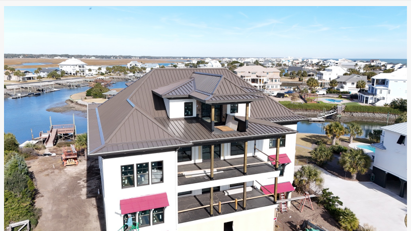
Showcasing the expert craftsmanship of Spann Roofing, captured beautifully by Splash Omnimedia.
