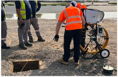
Electro Scan's ES-400 at work for a Middle East client that no longer uses CCTV images to prioritize repairs and rehabilitation decisions.
