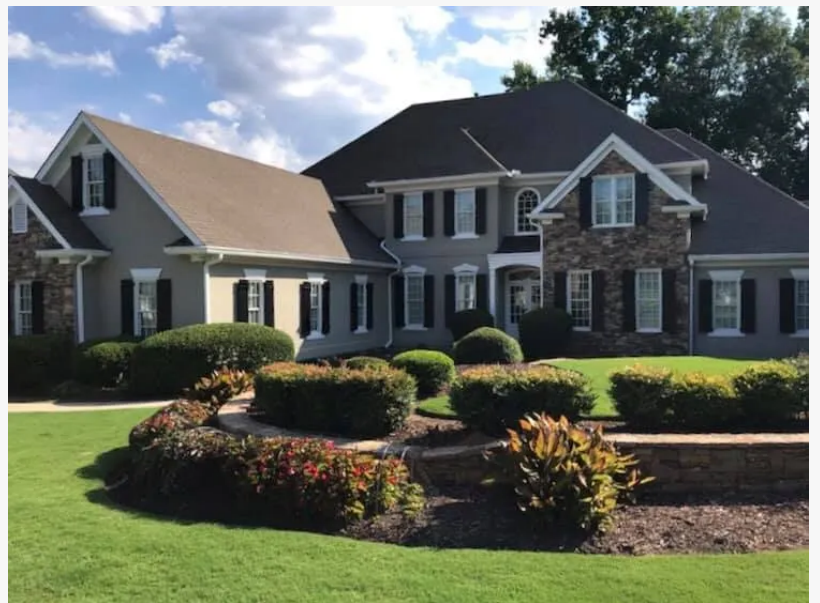
Residential Exterior Stucco Waterproofing
