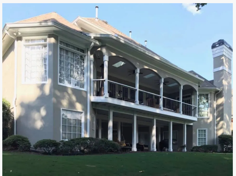
Residential Stucco Installation
