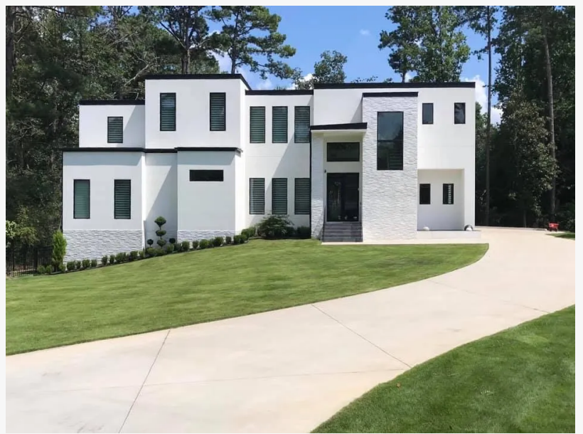
Residential Exterior Stucco
