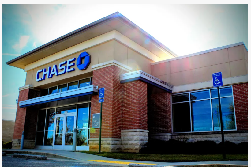
Commercial Exterior Stucco
