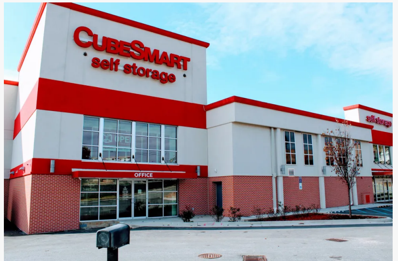
Commercial Strip Mall Exterior Stucco
