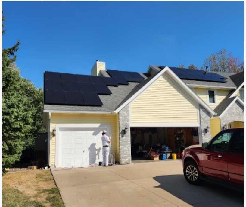
Wolf River Electric Residential Solar Completed
