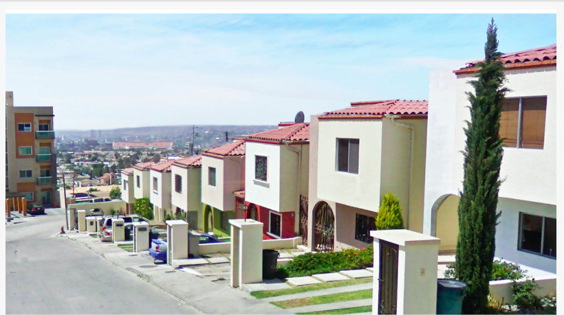
Casas Incablock BotBlocks, Ermita Sur - Tijuana, BC
