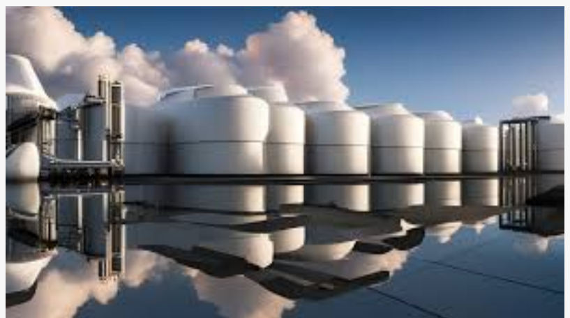
Hydrogen Energy Storage
