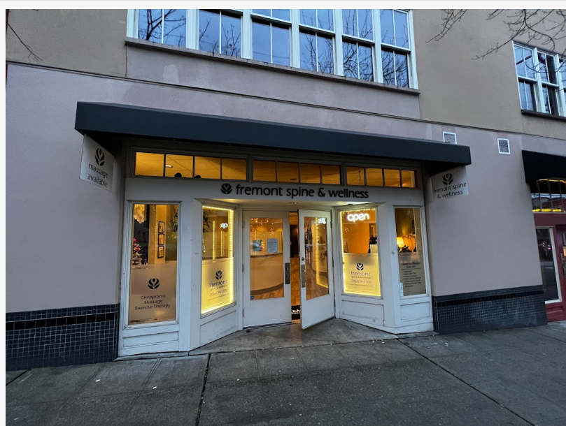
Fremont Spine + Wellness Building Exterior
