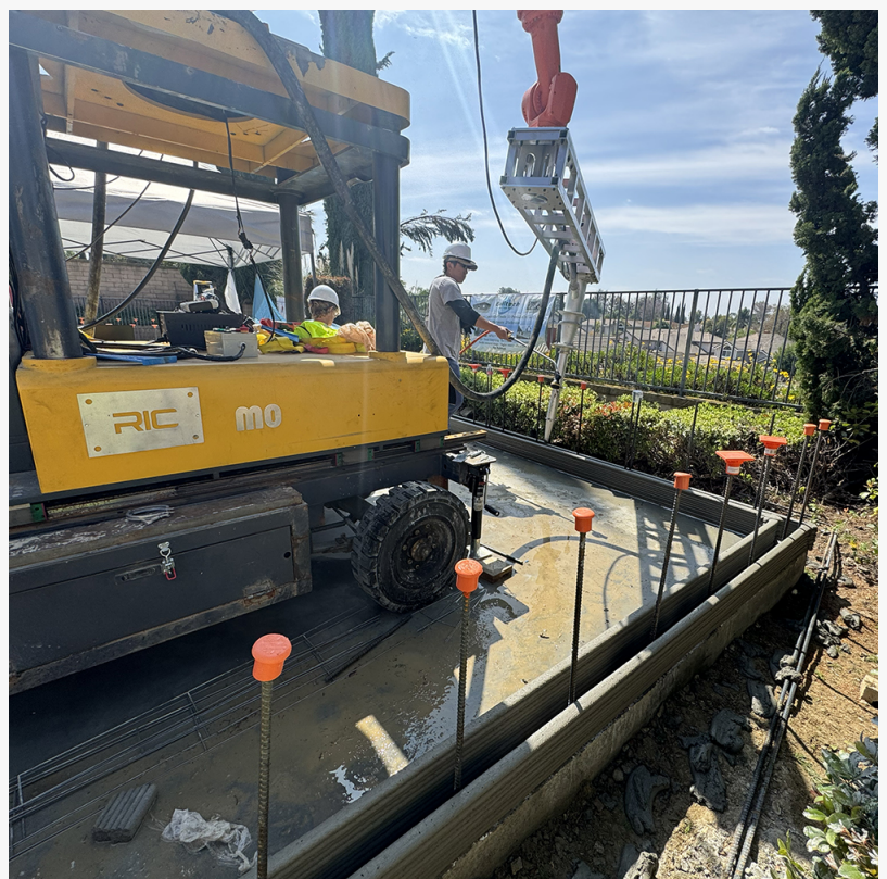
RIC Technology's robot 3D printing
