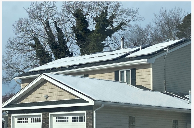
Snow on Solar Panels
