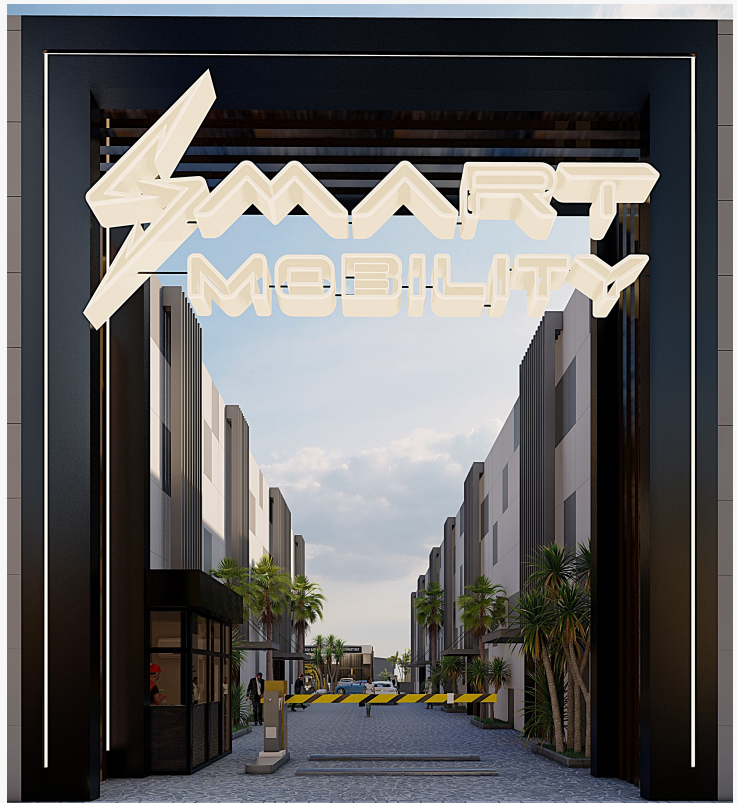
Smart Mobility International NEV Service Centre - Front Gate
