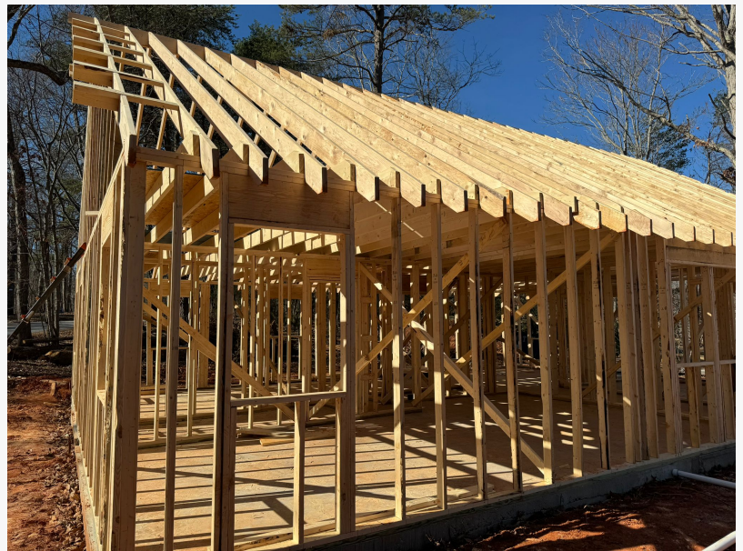
Custom home project by Garcia's Construction LLC
