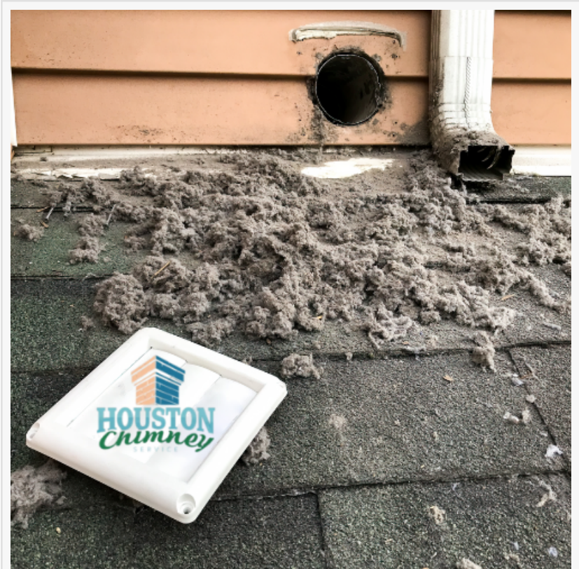
Expert duct and dryer vent cleaning by Houston Chimney Services, ensuring a safer, cleaner home environment
