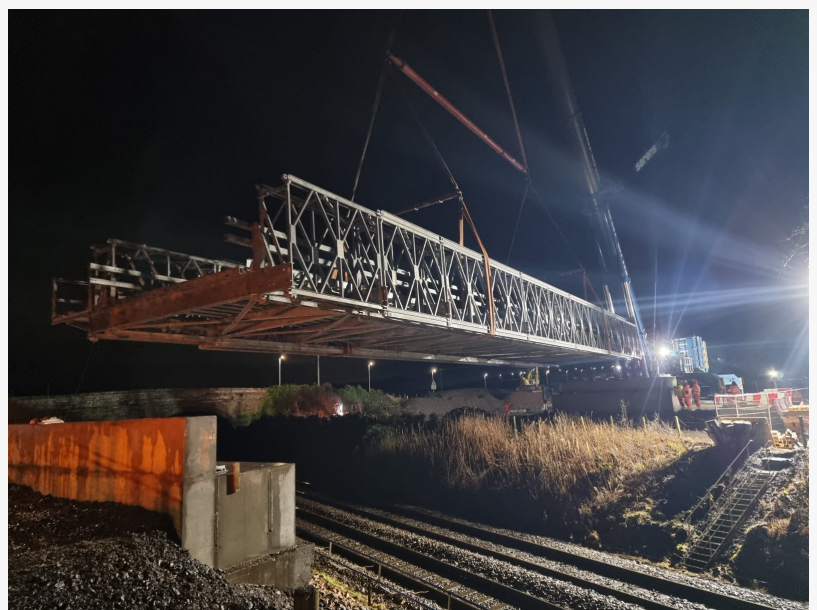
Overnight Installation of Acrow Temporary Bridge - Craigo, Scotland
