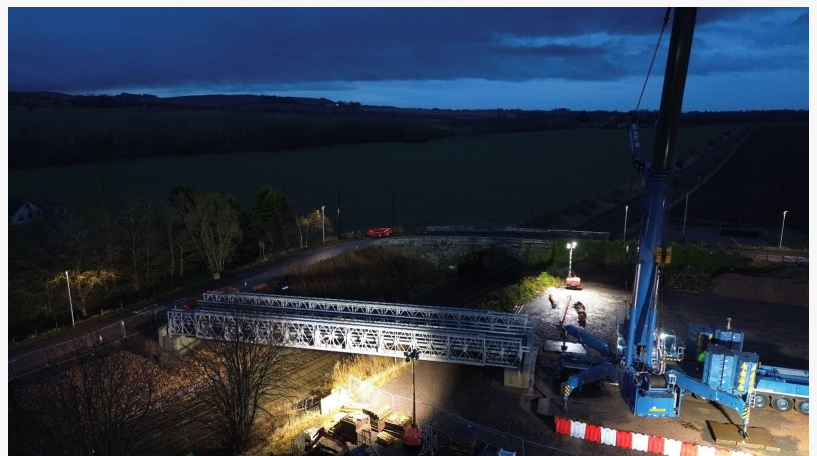
Overnight Installation of Acrow Temporary Bridge in Craigo, Scotland
