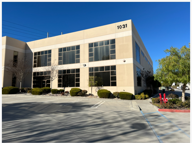
Aquacycl's new warehouse. Photo credit: Aquacycl.
