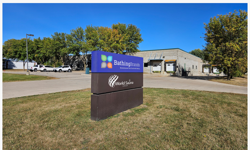
Hutchinson, MN Custom Sauna Facility
