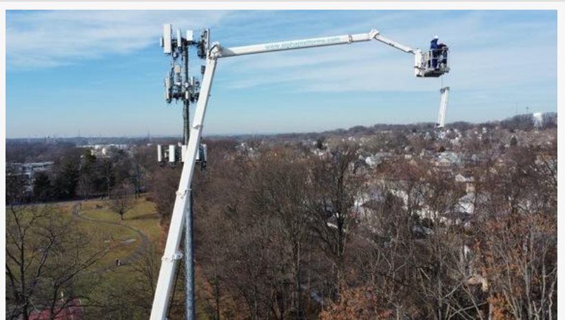
Alpha Platforms Lifting An Antenna
