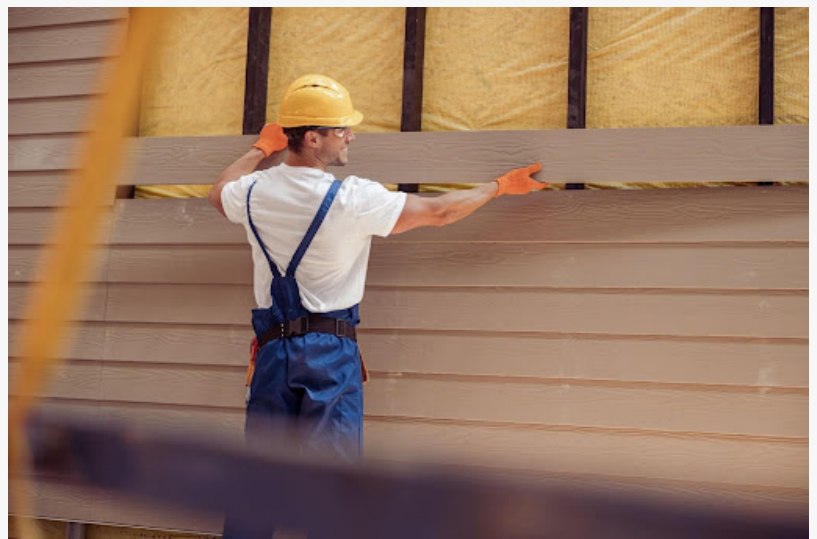
A male construction worker installing siding on a cabin.
