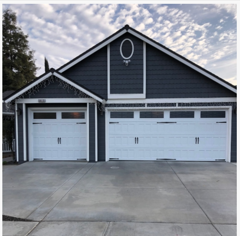
Larry's Garage Door Repair Installed New Garage Door
