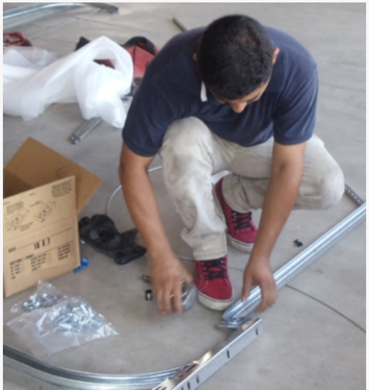
Larry's Garage Door Repair Team Working
