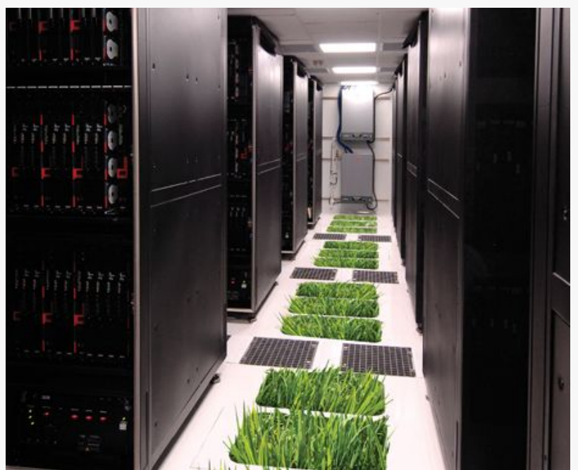
Green Data Center Market
