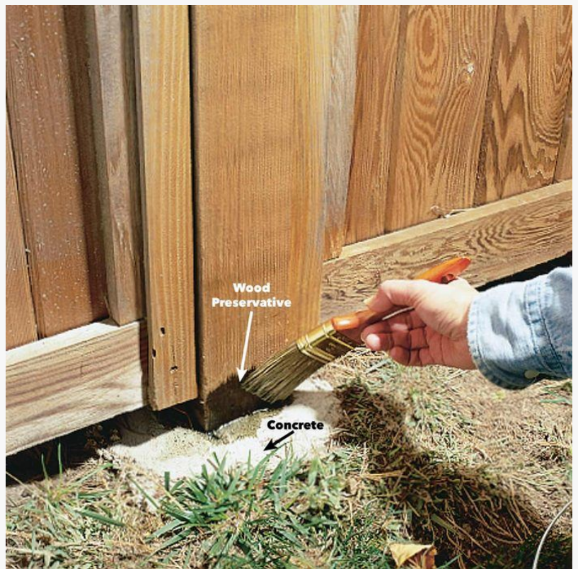
Fence Repair - Handyman Can Help
