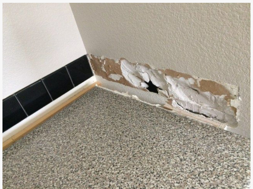
Dry wall - Handyman Can Help
