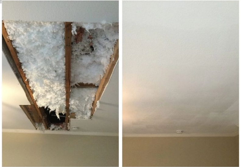
Ceiling Repair - Handyman Can Help
