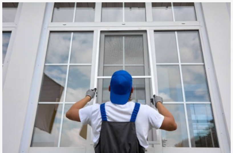
Window Installation - Handyman Can Help
