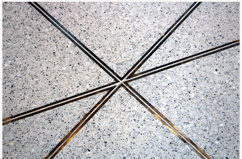
INTRICATE TRIANGULAR floor patterns in The Connector required nearly 2.5 miles of double zinc divider strips, precisely mitered to form complex geometric intersections.
