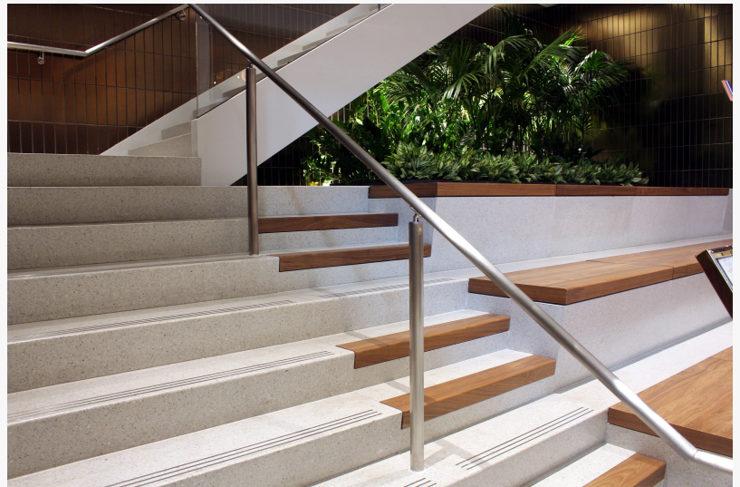
THE TERRAZZO installation at Winthrop Center includes seating steps crafted by the contractor.
