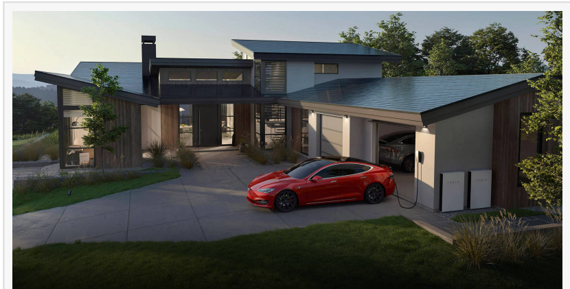
Shamrock Roofing and Construction Solar Installers
