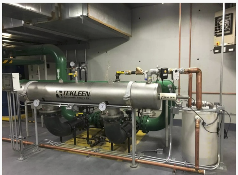
Tekleen Automatic Self Cleaning Filter At Wacker Drive, Chicago
