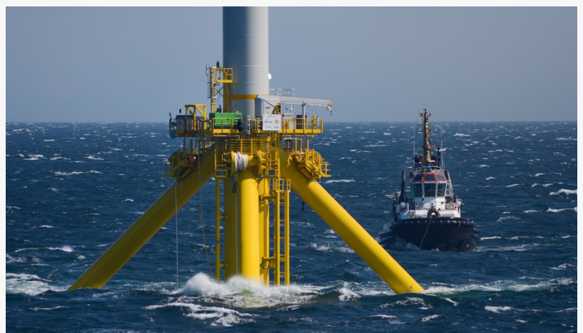
Global Offshore Mooring Systems Market
