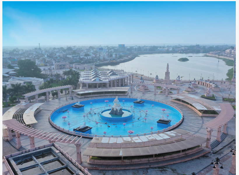
Aerial View of Mahakal Lok
