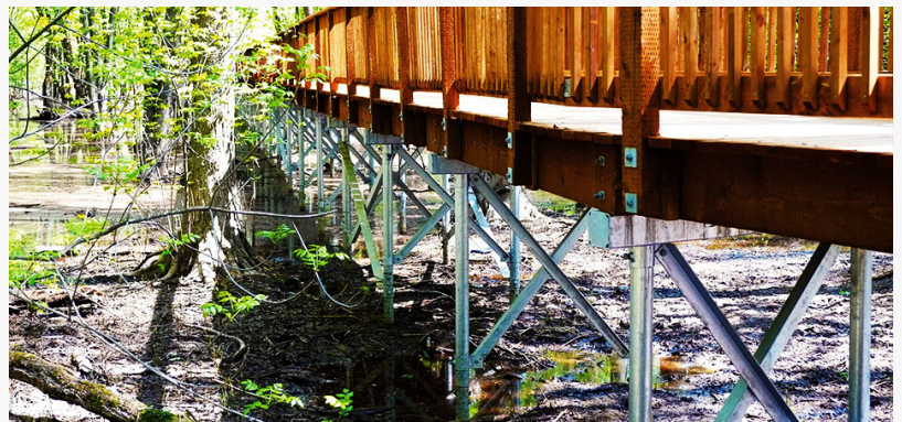
Recent Boardwalk Installation in Colorado
