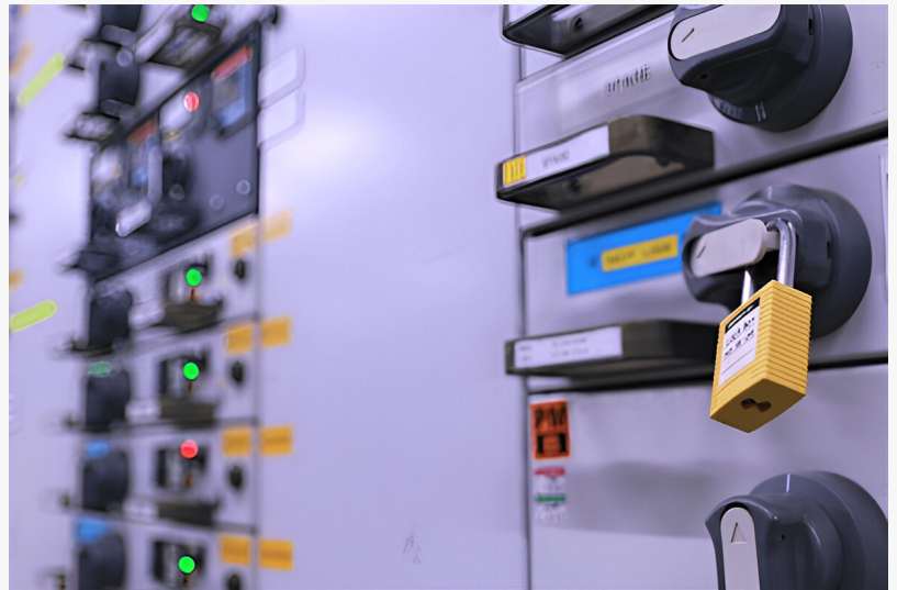
lockout tagout safety training-
