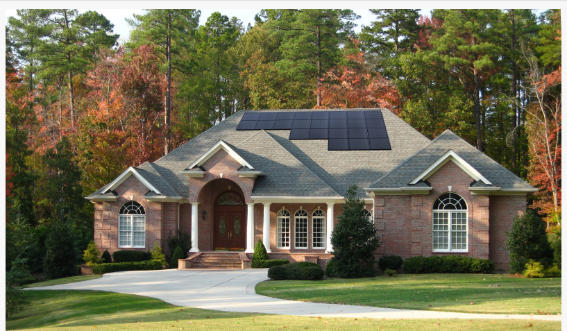
WRE REC Installation on 1-story Brick Home
