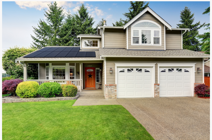
WRE REC Installation on 2 Story Home
