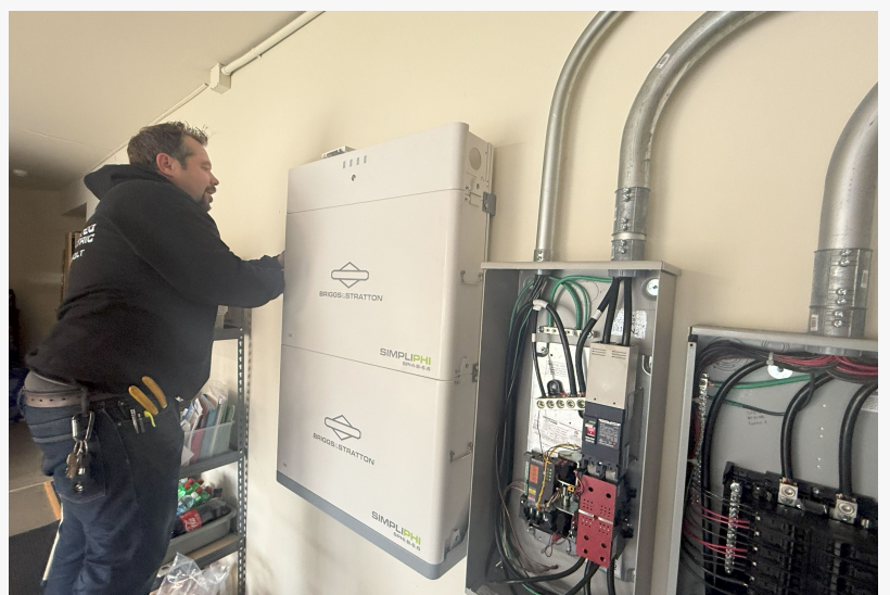
Our lead technician Jesse installing a sleek, reliable battery backup system
