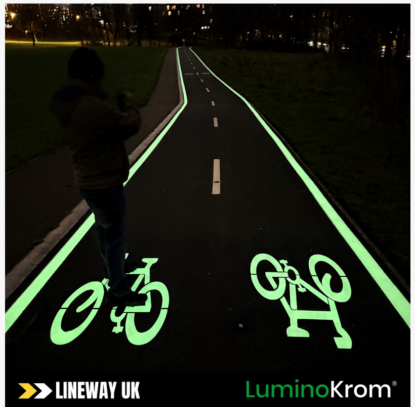
Glow-in-the-dark line marking paint at Everton Park
