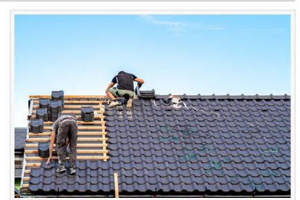
Craftsmen perform storm damage restoration services, building a new roof from ceramic tiles to ensure durability and weather resistance.
