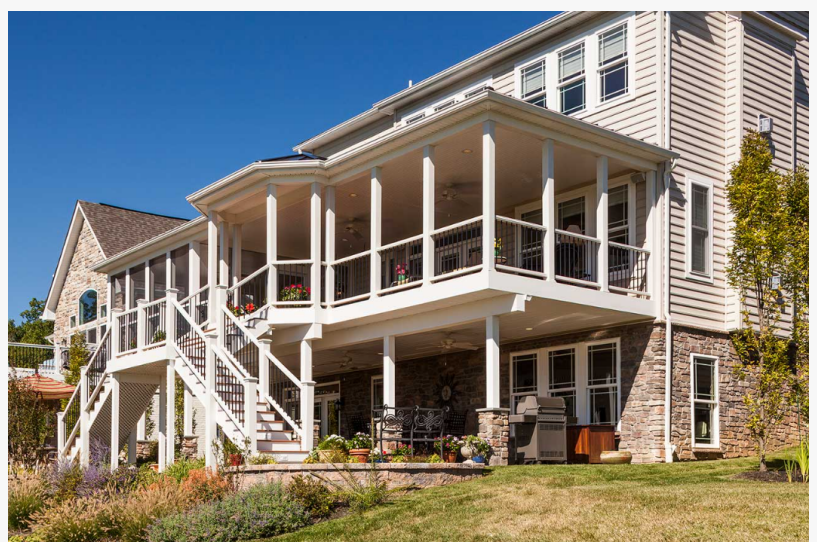
T.W. Ellis Home Porch Addition
