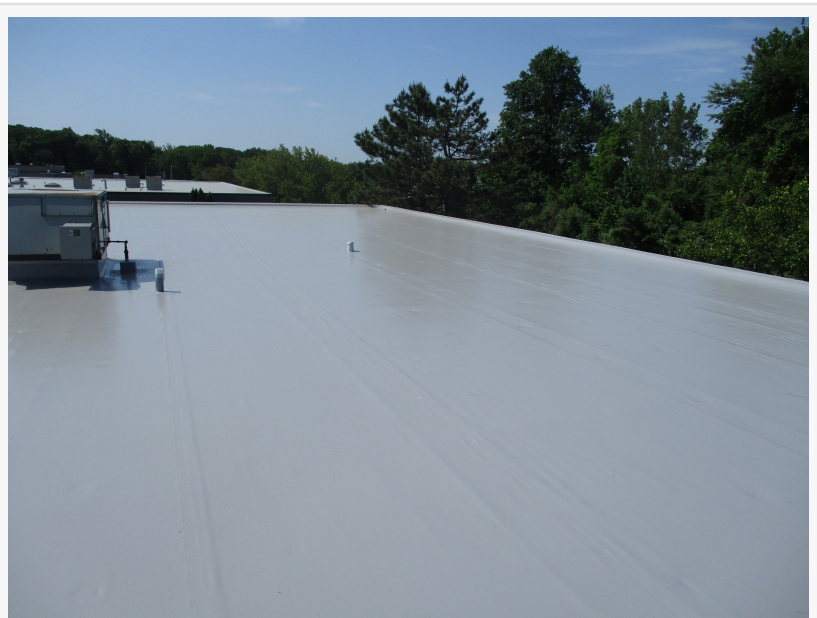
Completed PVC grey roof
