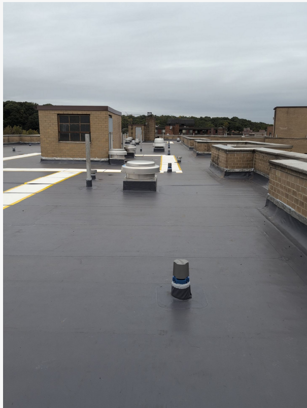
Flat roof with walkpads
