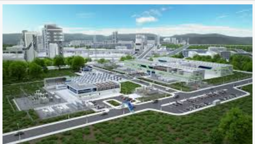
Data Center Substation
